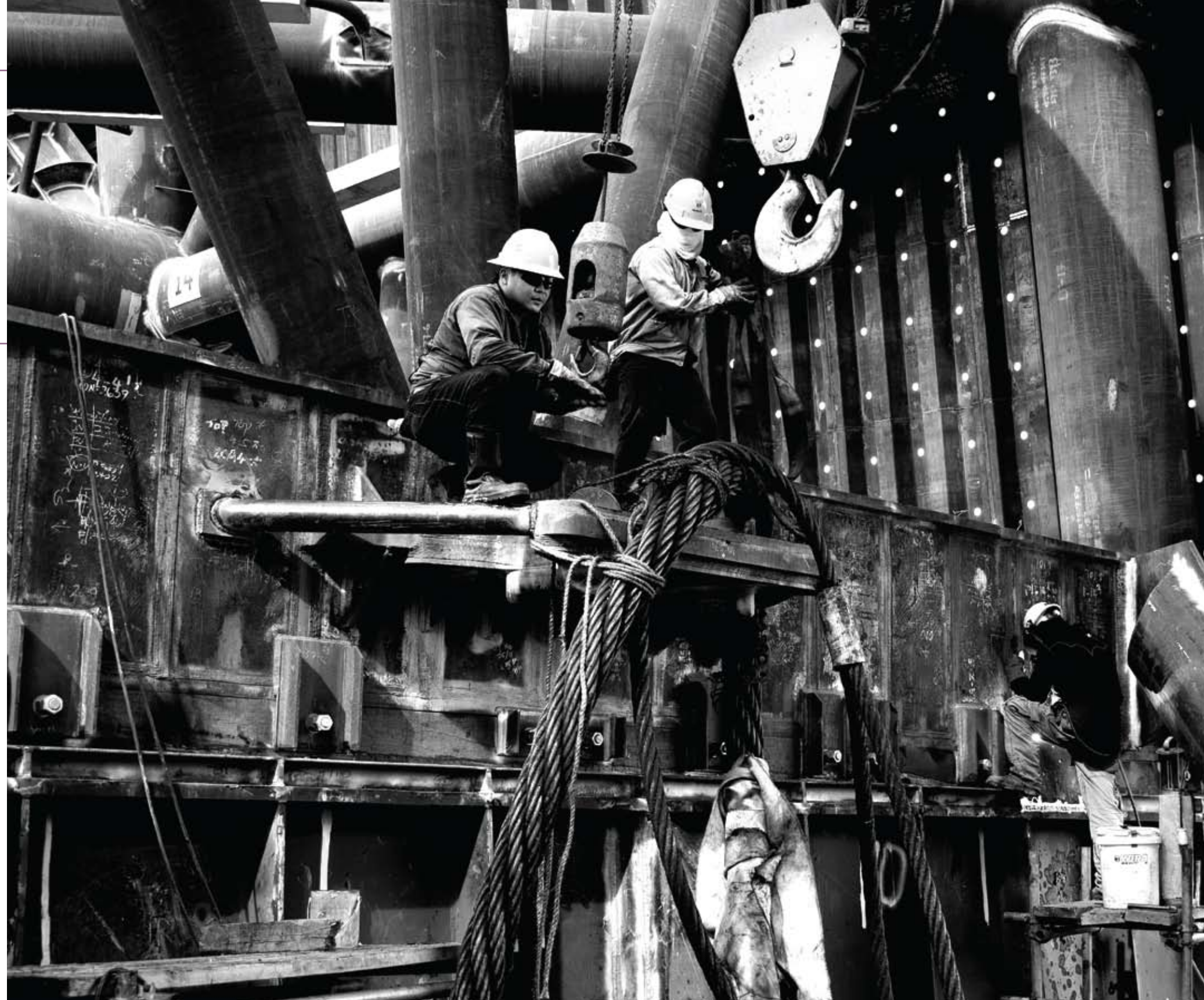
Installing a steel jacket for a facility in the oil and gas industry.
